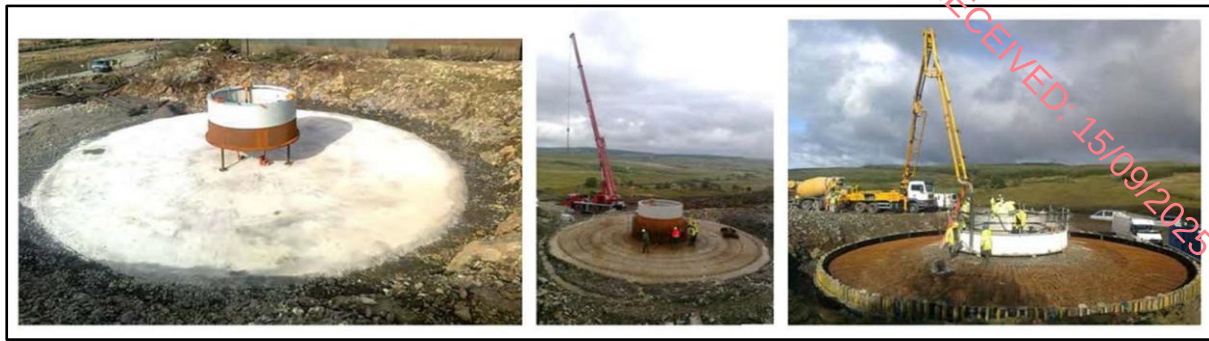
Figure 2-13: Turbine Foundation, Steel Reinforcement and Concrete Pour
